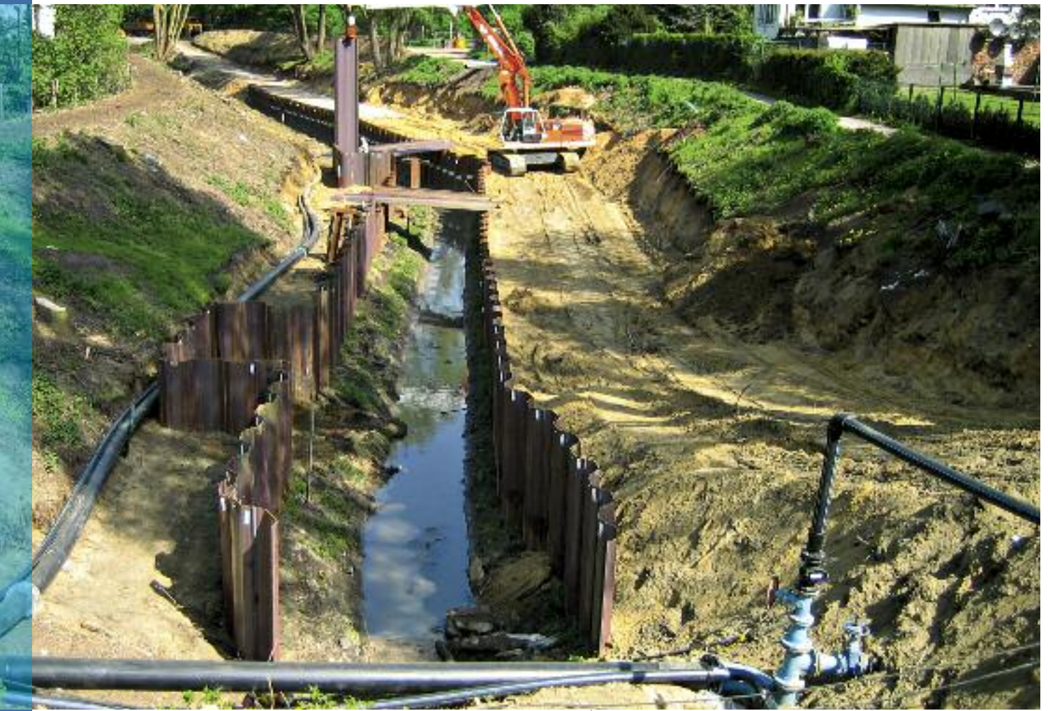
Sustainable building project: Effective groundwater drainage through sheet piles in a body of water.
