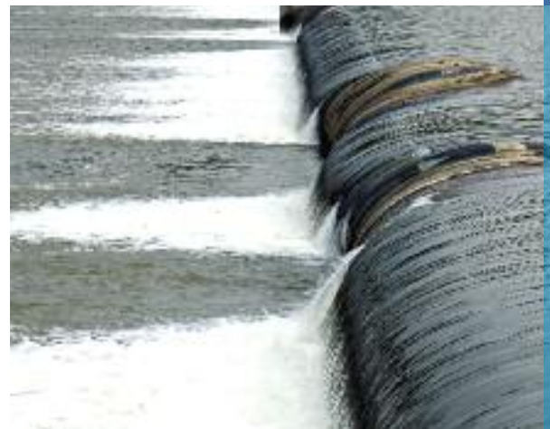
Weir for regulating the water level of the river: Effect on the proportion of bank filtrate of a water catchment.
