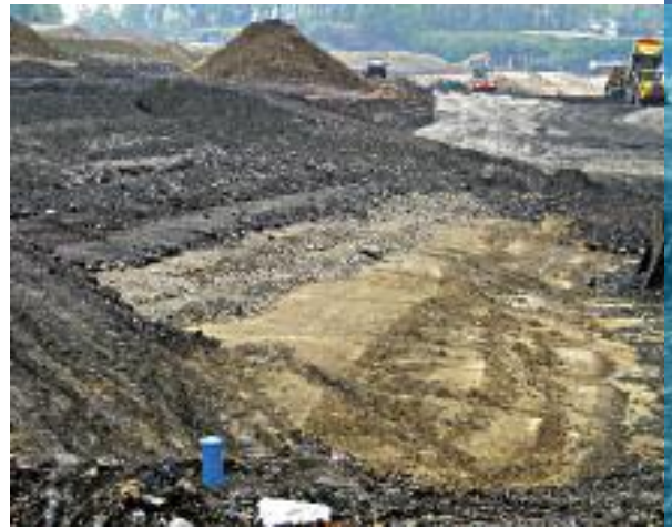
Building a "city lake": Groundwater monitoring as important element of the construction stage.
