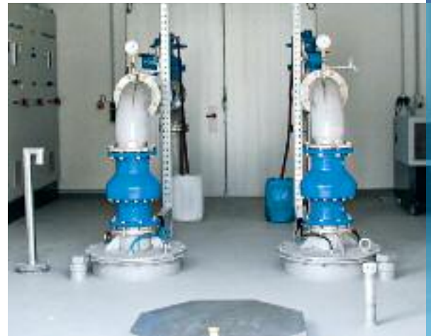
Efficient water catchment: Pump installation of groundwater catchment in a waterworks.
