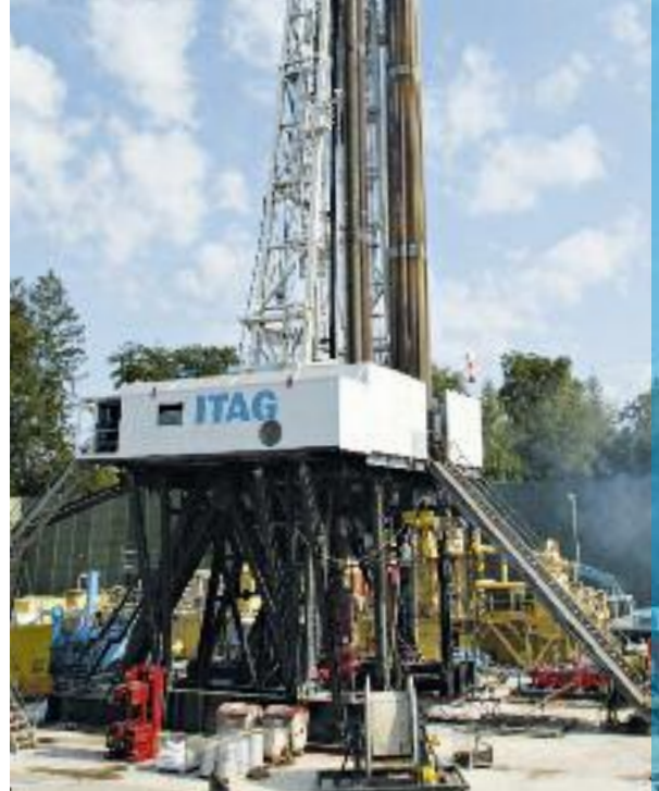
Exploration measure: drilling a geothermal well in maximum depth.
