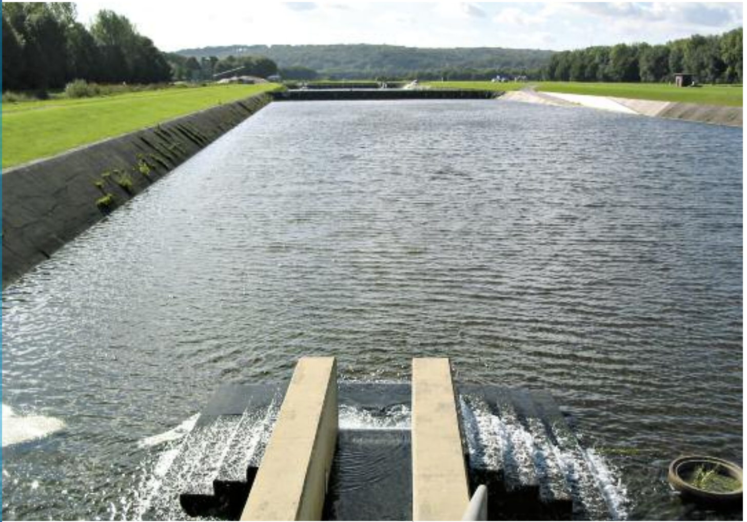
Seepage reservoir: groundwater recharge through infiltrating bank filtrate.
