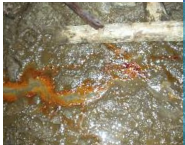
Redevelopment action required: Flooding and discharge of seepage water in a uranium mine.
